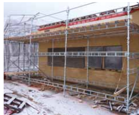
Stabilt underlag for murerstillads
