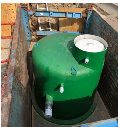
Installationsbrønd type D.
