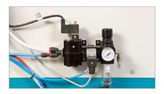
This alarm appears if there is too little air pressure in the machine. Check the air supply.
