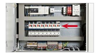
The motor protection switches for the scraping roller motors are located in the middle electrical cabinet. If a red button is "in", then the motor has cut out. Press the black button in if the motor protection switch has cut out.
