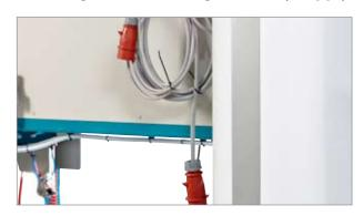
The machine uses two plugs: a 32 A CEE plug and a 16 A CEE plug for connecting a 3 x 400 Volt power supply with neutral (N) and earth (PE) conductors. The ground fault circuit breaker (HPFI) for the 32 A plug must be approved for frequency converters.
