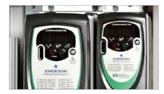
One of the frequency converters has cut out. Check whether there is a fault in the sawdust dispenser motor or the beam driver. Press <Emergency stop> and wait 30 seconds before resetting the error.
