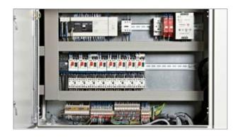
The middle cabinet contains the motor protection switches for the eight scraping rollers. From left to right, these switches protect the following motors:
