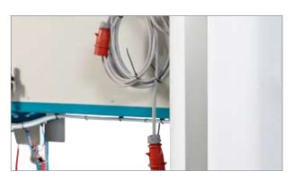
The machine is fitted with two plugs: a 32 A CEE plug and a 16 A CEE plug for connecting a 3 x 400 Volt power supply with neutral (N) and earth (PE) conductors. The ground fault circuit breaker (HPFI) for the 32 A plug must be approved for frequency converters.
