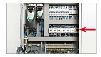
The motor protection switch for the fat pump is located in the electrical cabinet to the left. Press the black button in if the motor protection switch has cut out.
