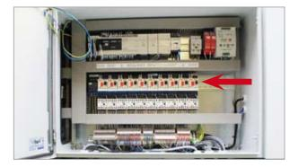
The motor protection switches for the scraping roller motors are located in the middle electrical cabinet. If a red button is "in", then the motor has cut out. Press the black button in if the motor protection switch has cut out.
