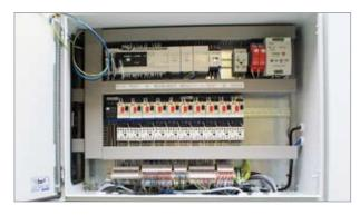
The middle cabinet contains the motor protection switches for the ten scraping rollers. From left to right, these switches protect the following motors:
