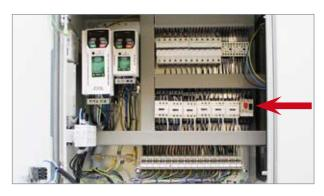
The motor protection switch for the fat pump is located in the electrical cabinet to the left. Press the black button in if the motor protection switch has cut out.
