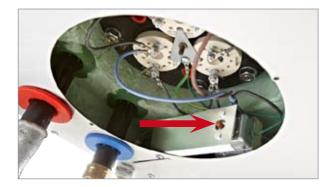
If the container's overpressure fuse cuts out, you will need to remove the cover from the base of the water heater and press the red <Reset> button.
