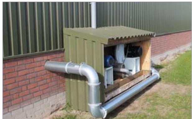
The fan makes a lot of noise and should therefore be placed in an adjoining, sound-proofed room, or outdoors. If the fan is placed outdoors, make sure to position it in a sheltered location to protect it against rain, etc.
