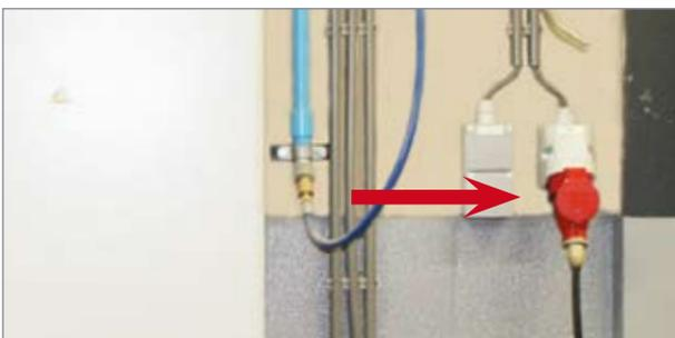
The system is to be connected to a 3 x 400 volt power supply with neutral (N) and earth (PE) conductors, and protected with a min. 32 A, category C fuse. Connect the system to the power supply with a CEE plug or a supply separator, so that it is easy to disconnect the power for maintenance procedures and repairs.
