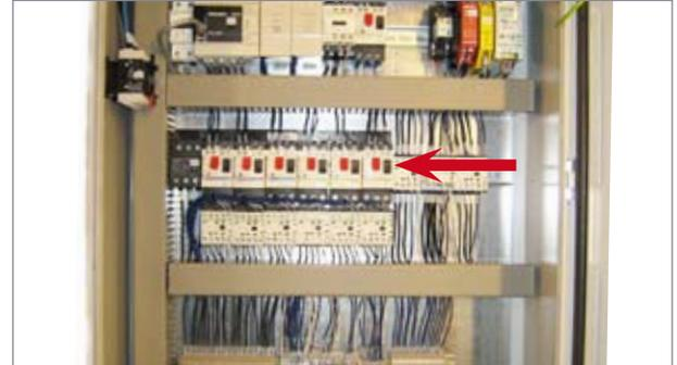
One of the system motors has overloaded. It may be the motor for one of the four drums, for the fan or for one of the drive stations (sawdust).
