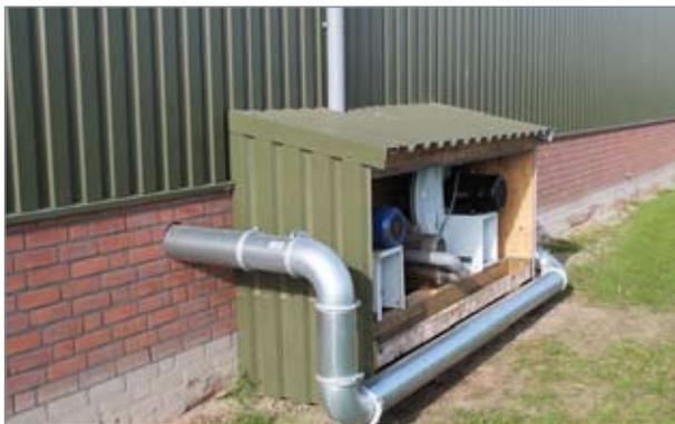
At the end of the first day using a new fan, all the screws must be checked and tightened. They must, of course, be kept tightened at all times subsequently.
