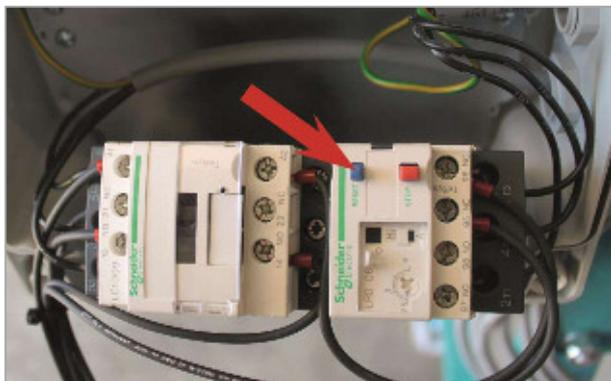
The panel contains the motor protection that protects the motor from overload. If the motor protection has tripped, open the panel via the four corner screws and reactivate by pressing the blue button.
