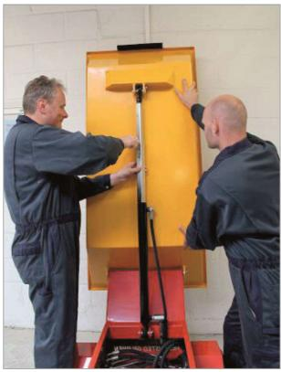
While one person holds up the tray, the other mounts the safety fitting on the hydraulic cylinder.
