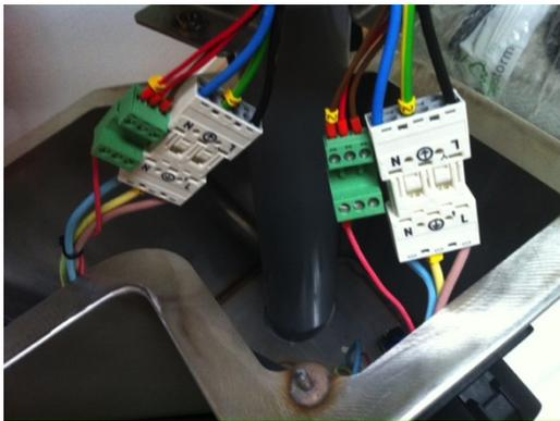
3. Finally tighten the screws in the bottom.
