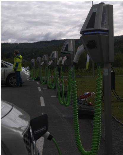
Figure 2 Example of pole mount installation
